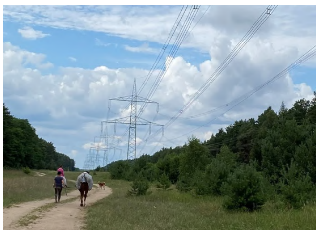
Locals walk along a grid corridor that benefits from IVM, 2023. Photo: ©50Hertz Transmission GmbH
