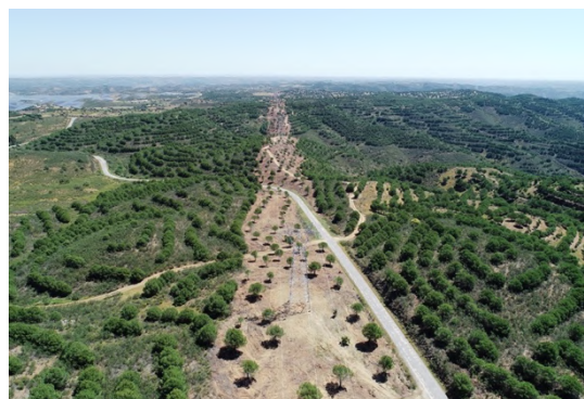
Grid corridor with the placement of trees that fulfils Portuguese fuel management criteria, 2024. Photo: © Redes Energéticas Nacionais - REN
