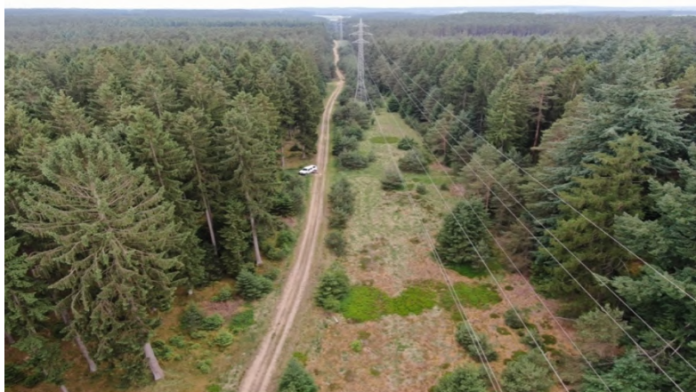
Perspective view of a grid corridor with well-maintained forest edges, 2023. Photo: ©E.ON SE
