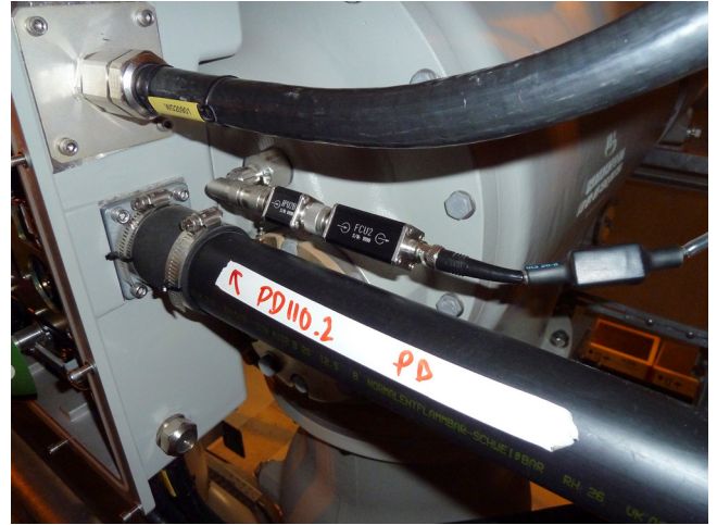
Figure 1: Horizontal sensor connection with use of N-N-Adapter and 90° angle connection at an ABB indoor GIS
