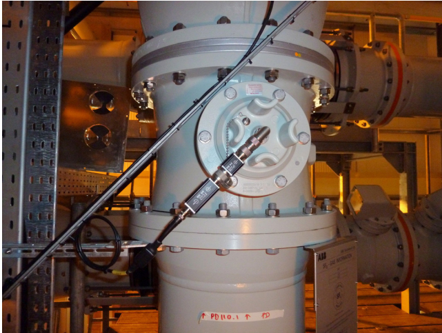
Figure 1: Horizontal sensor connection with use of N-N-Adapter and 90° angle connection at an ABB indoor GIS
